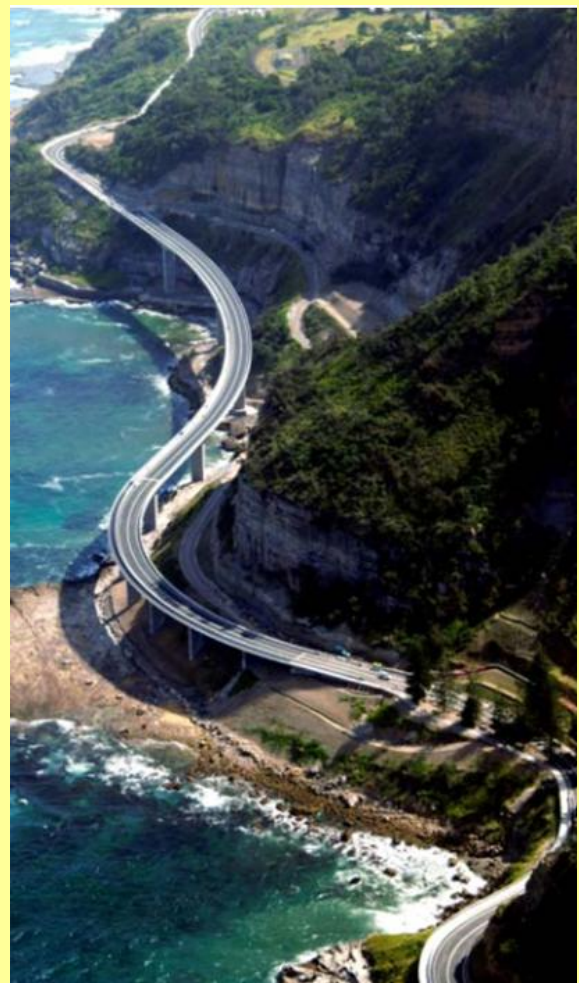
Pacific Coast Highway in Australia. Replacement of one of the most dangerous section. Existing highway had to remain functional while new highway was built.
